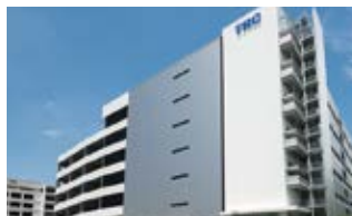
2018 Relocates and integrates Tokyo Logistics Center
